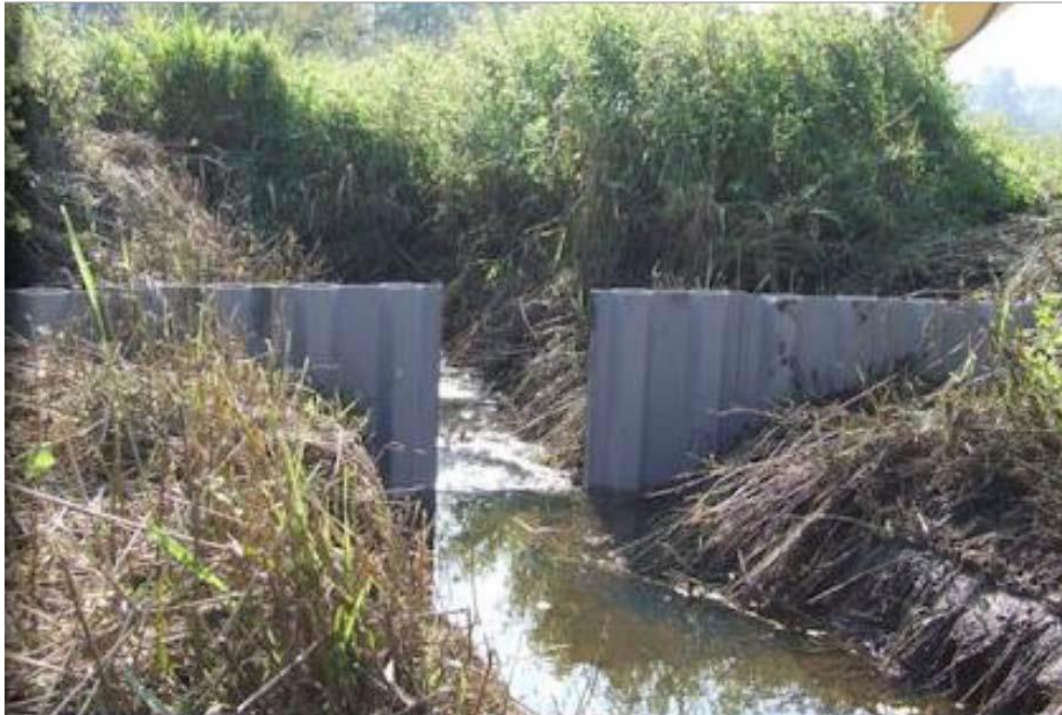
Plate 4-38 Partially blocked drain, with level of blocking determined by driving plastic piles in the centre of the drain further into the peat (Source: NPWS, 2017). Such measures will ensure a rise in the water table while not creating open waterbodies.
