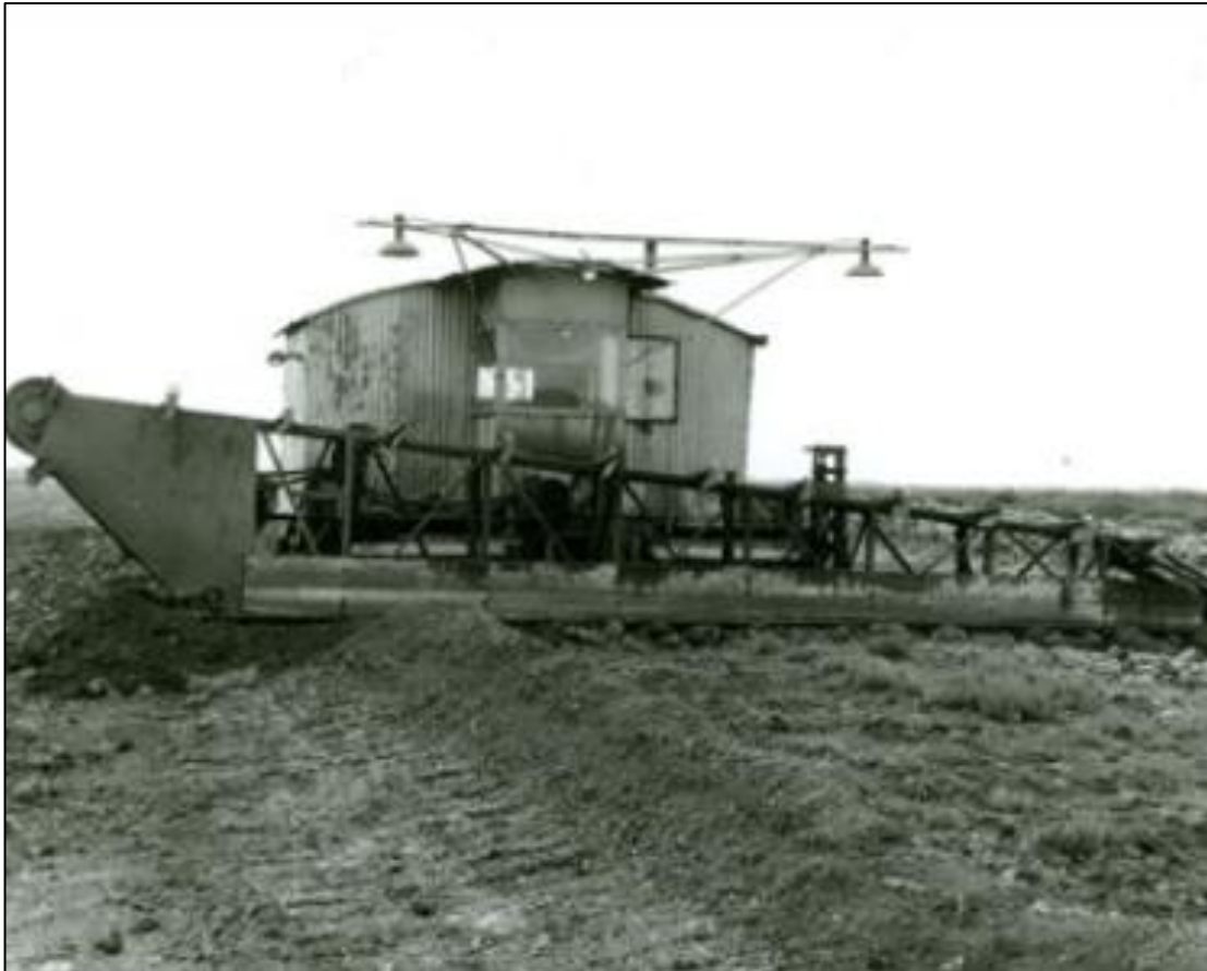
Plate 4-6 Levelling Machine Type – Scraper. Source: https://www.bordnamonalivinghistory.ie/equipment-detail/levelling-machine/
